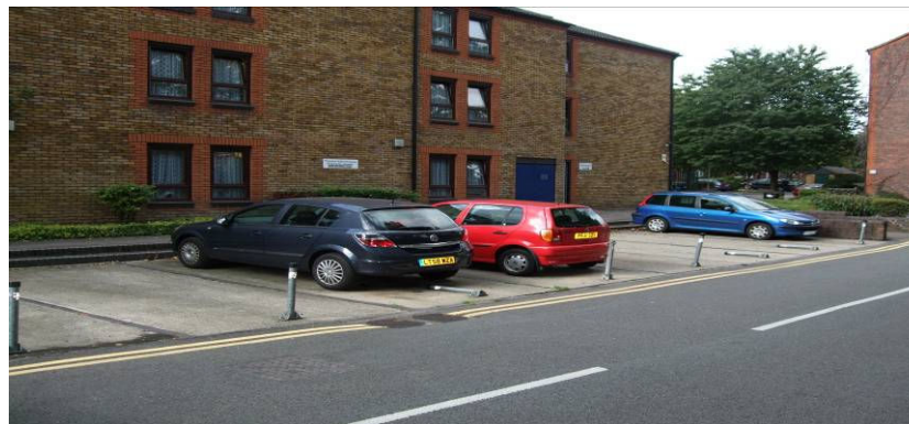
Drop Down Bollards at Hartington Close
